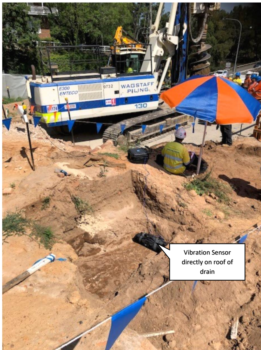
Figure 1 Test Pile Monitoring
