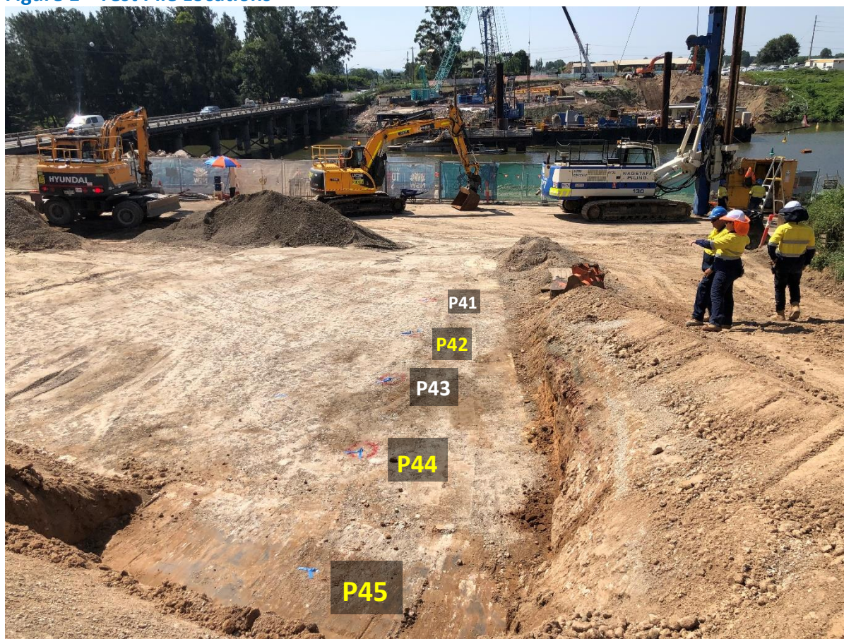
Figure 1 Test Pile Locations
