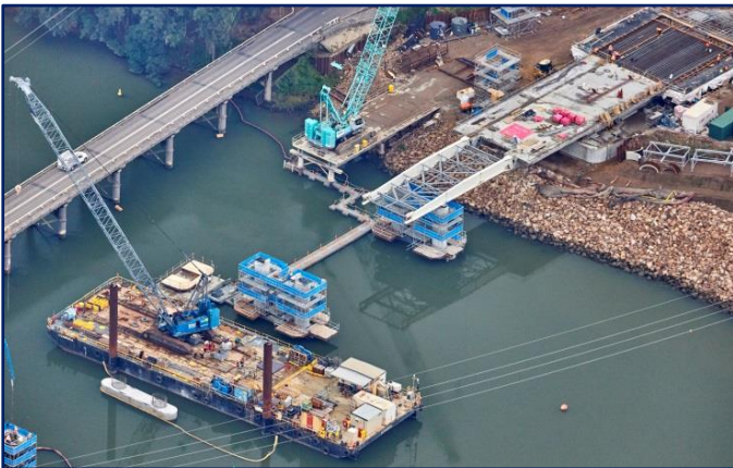
Work to launch the bridge deck continues
