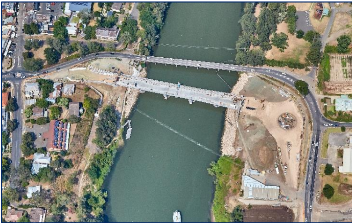
Aerial view of construction progress
