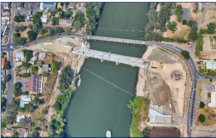
Aerial view of construction progress
