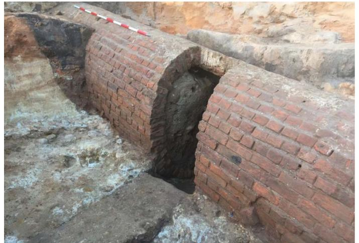
*Brick barrel drain (showing 1930s sewer work damage) to be preserved in its current location*
