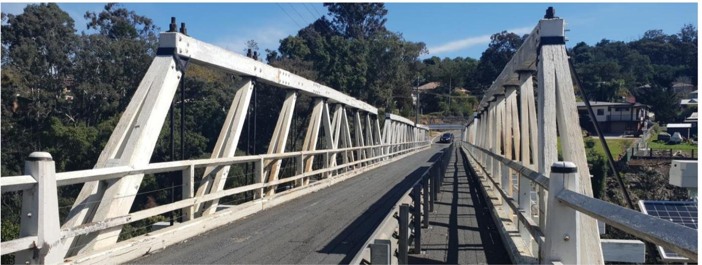
Victoria Bridge upgrade Stage 1 – the solid timber top chords providing support for the bridge will be removed and replaced
