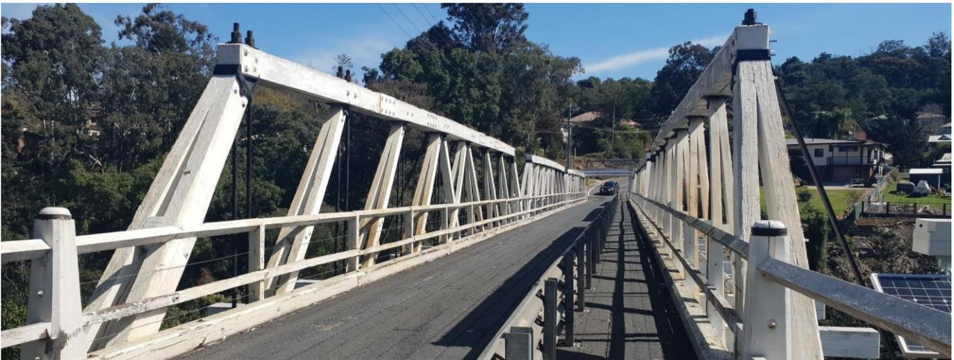
Victoria Bridge at Picton - in Stage 1 of the upgrade we will remove and replace the solid timber top chords that provide support for the bridge
