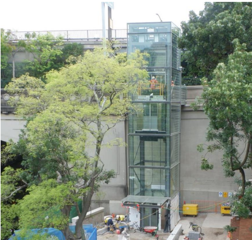
The southern lift on Cumberland Street, The Rocks
