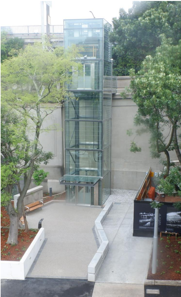
The Southern Lift on Cumberland Street, The Rocks
