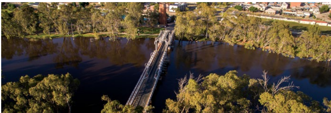
Swan Hill Bridge
