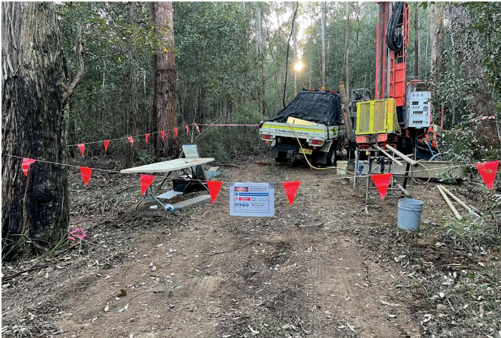
A geotechnical drill rig in operation along the corridor
