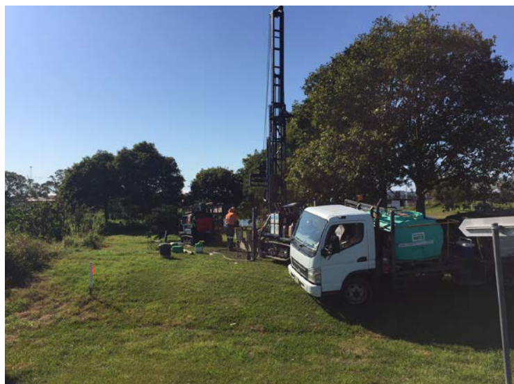
Drill used for geotechnical investigations (July 2015)
