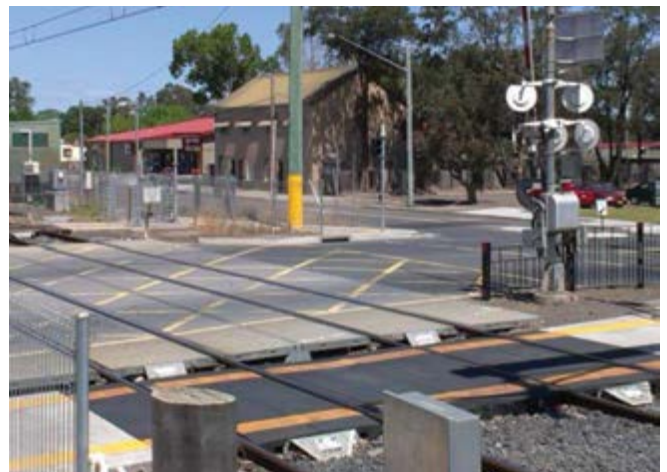
Level crossing on Garfield Road at Riverstone.
