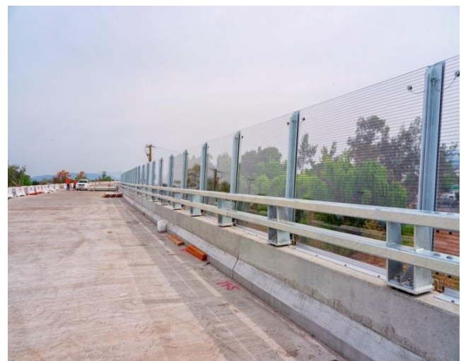
Completed noise barrier on the bridge over Parsons Gully
