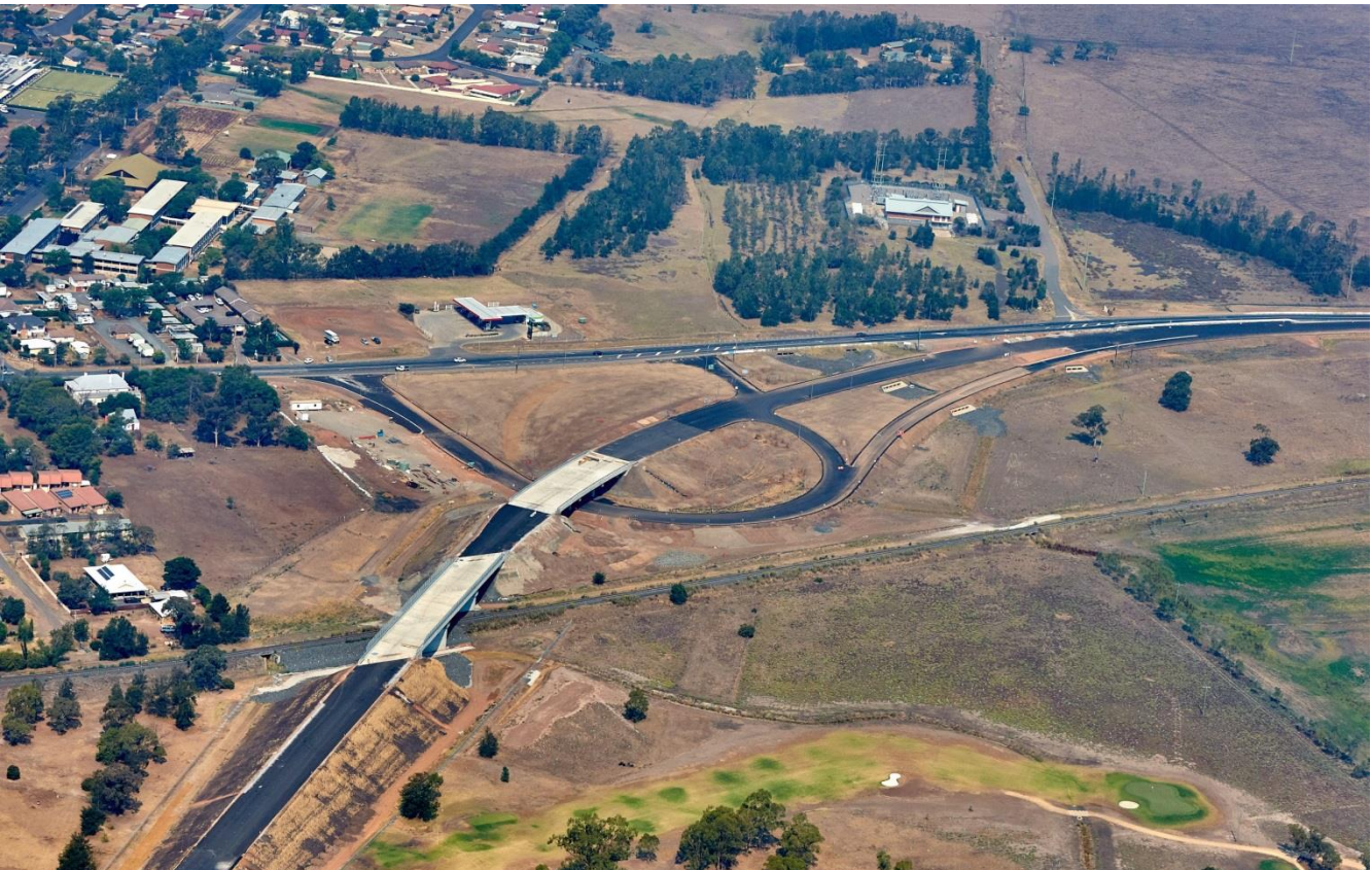
Really looking like a highway bypass: the view east over the southern interchange with the rail bridge and Kelly St bridge visible
