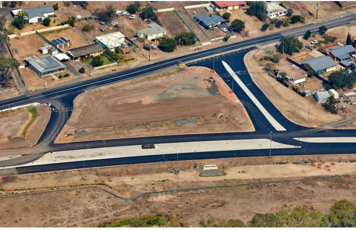
The northern intersection showing the existing highway at top
