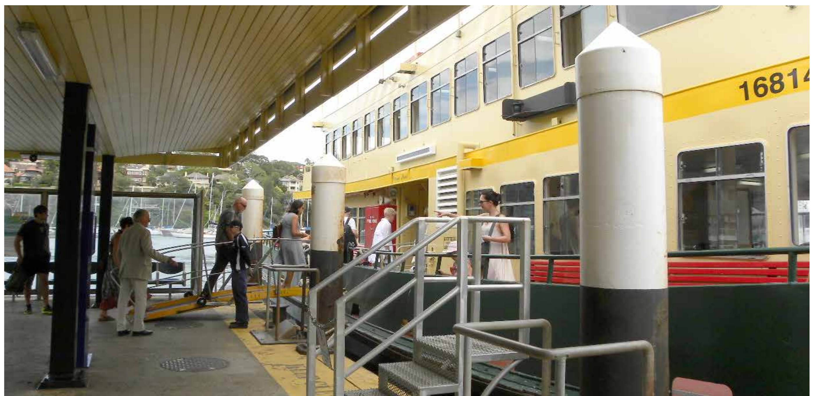
The existing Mosman Bay Wharf pontoon.
