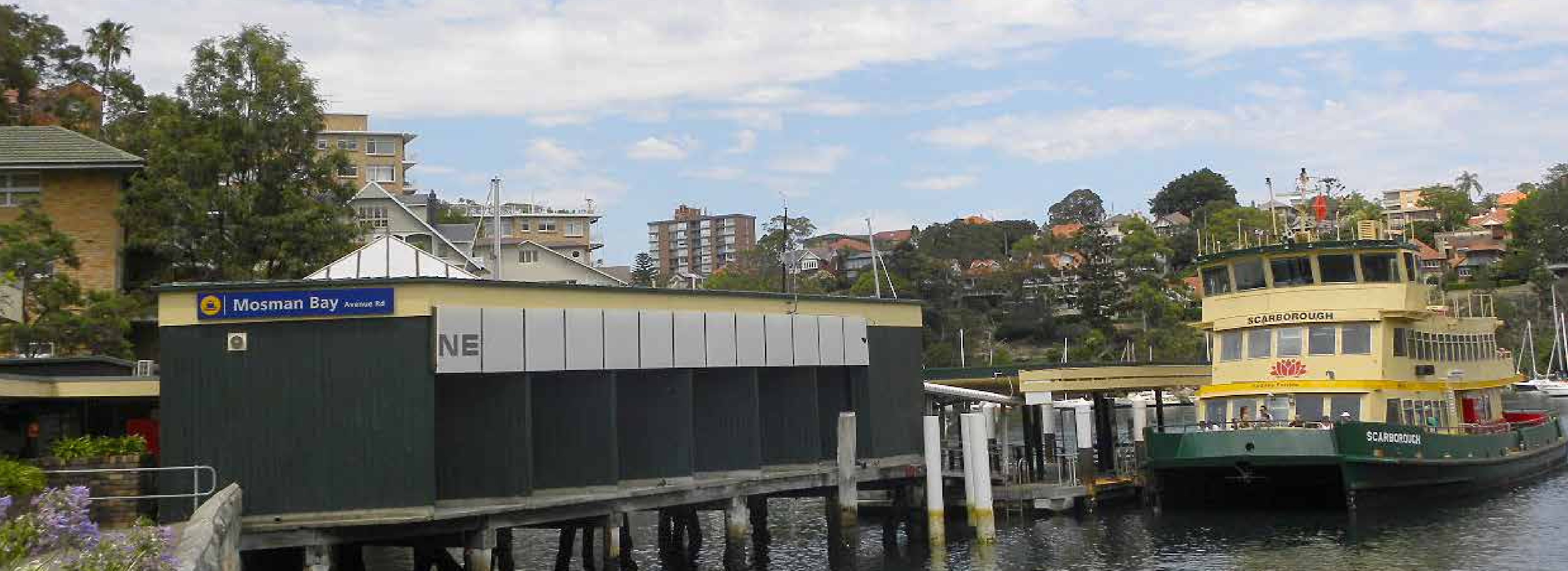
Existing Mosman Bay Wharf viewed from the land looking south east.
