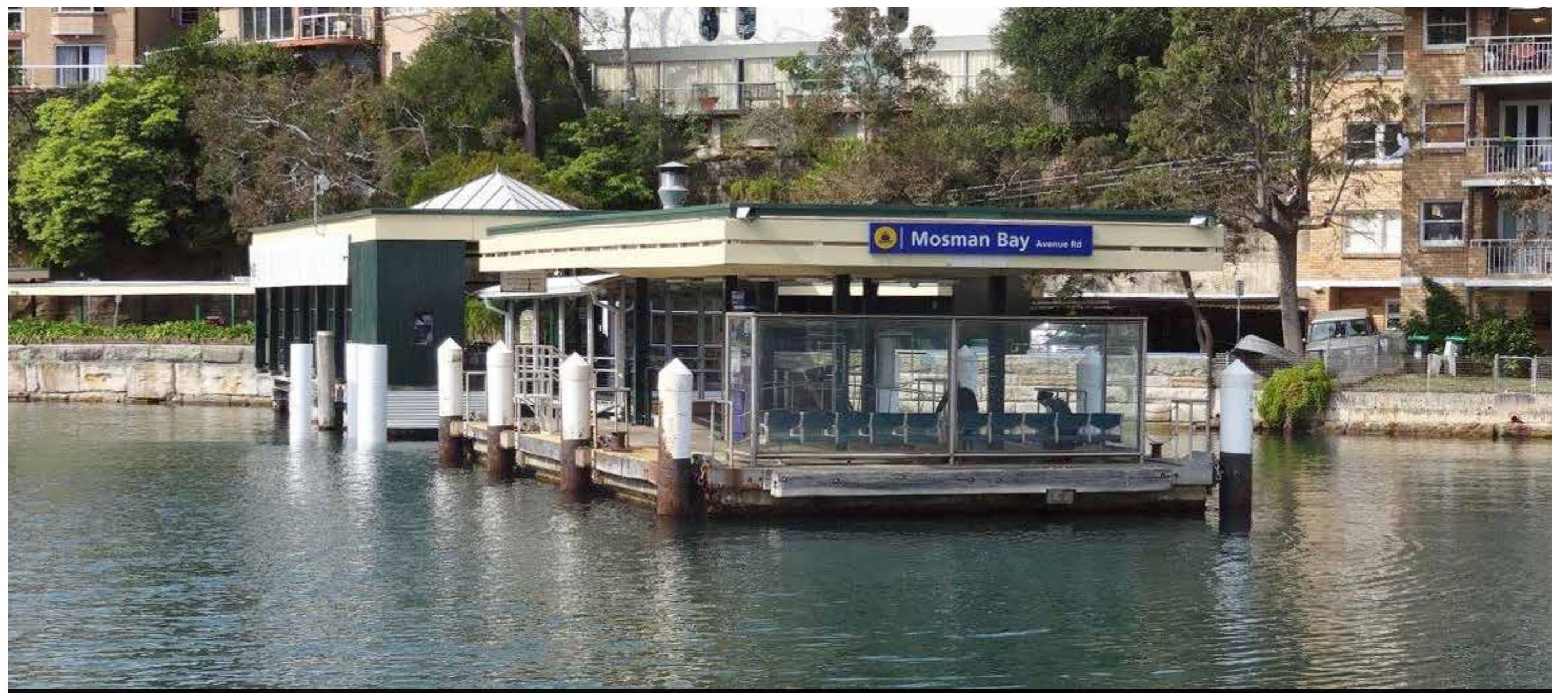
Existing Mosman Bay Wharf viewed from the water.
