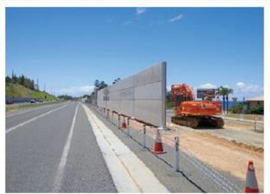
Photograph of similar noise walls being built on the Pacific Highway Sapphire to Woolgoolga upgrade
