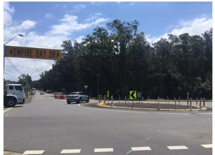
*The old roundabout and concrete medians have been replaced with a temporary asphalt roundabout and reflective markers while work is carried out*
