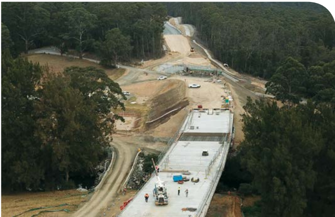
Construction work, Dignams Creek Bridge looking south
