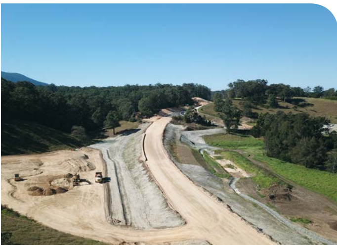
Looking north over the new alignment from near Dignams Creek
