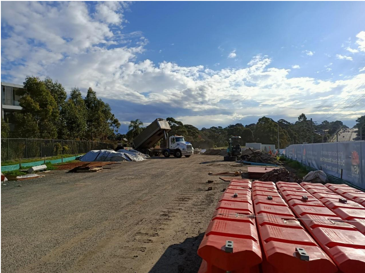
Site compound at 166a Epping Road, North Ryde
