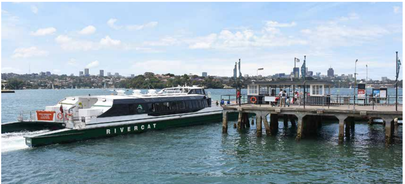
The existing Cockatoo Island Wharf
