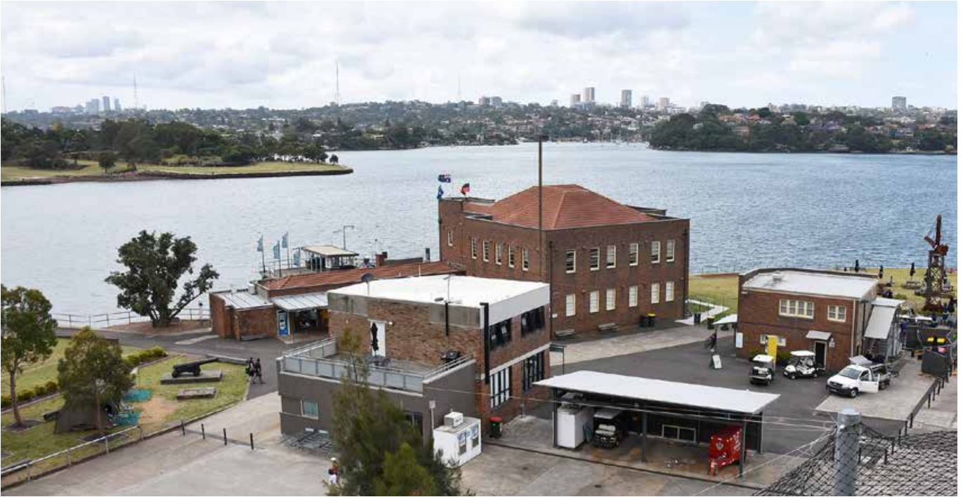
The existing Cockatoo Island Wharf
