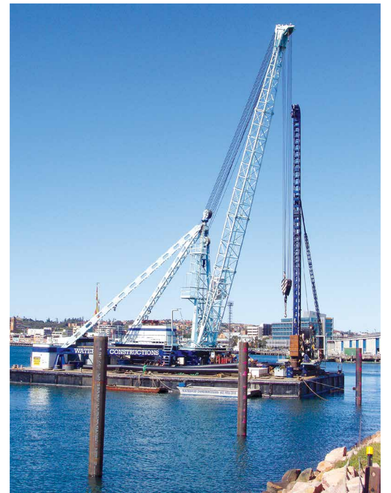
Barge-mounted cranes near a work site in Sydney Harbour
