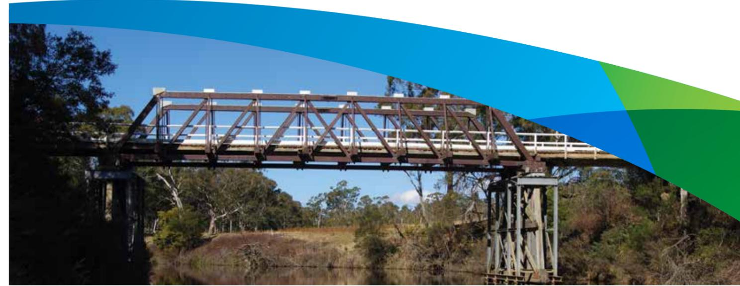
The existing Charleyong Bridge. Temporary steel supports are in place to support the bridge and approach spans.
