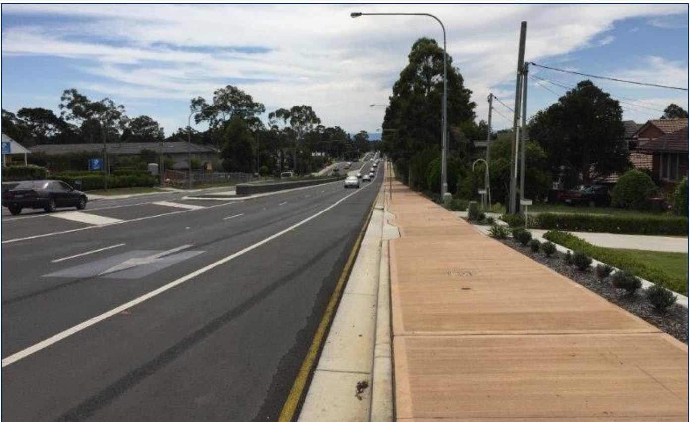
Completed section of Showground Road between Kentwell and Cecil Avenues
