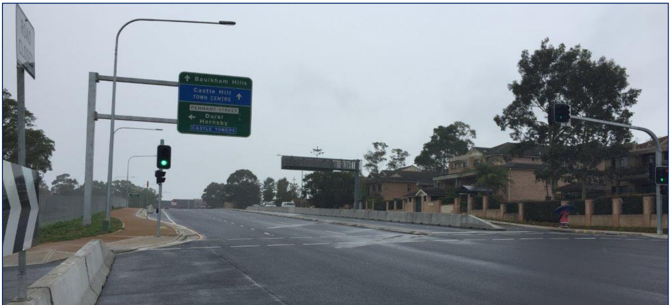
The newly upgraded Showground Road eastbound at Kentwell Avenue
