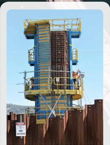
Formworkers and steelfixers worked hard to complete the cage and steel reinforcement at Pier 1 before the first pier arm concrete pour in November.
