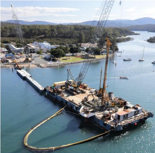
Concrete is pumped onto the river from the southern or northern foreshore. It is pumped through pipes and hoses placed along pontoons and barges across the water.
