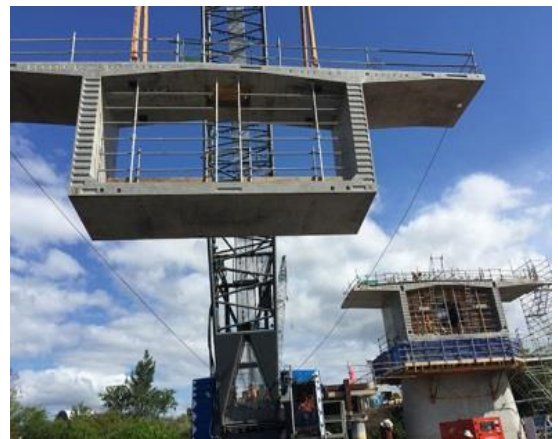
Concrete segments used on other Roads and Maritime projects
