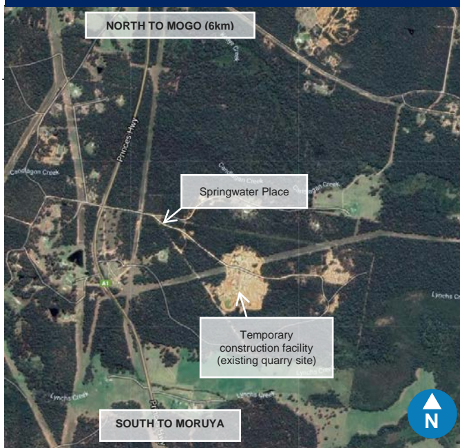
The pre-cast facility is located about 6km south of Mogo in an existing quarry site
