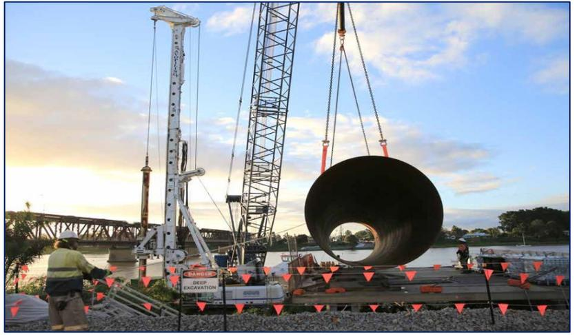
Piling materials being transported onto the river using a temporary jetty
