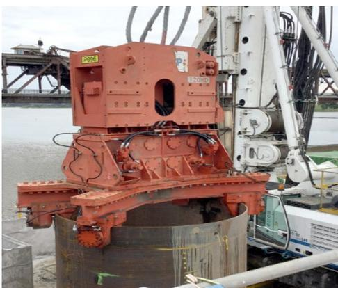
A piling hammer vibrating a steel casing into place.
