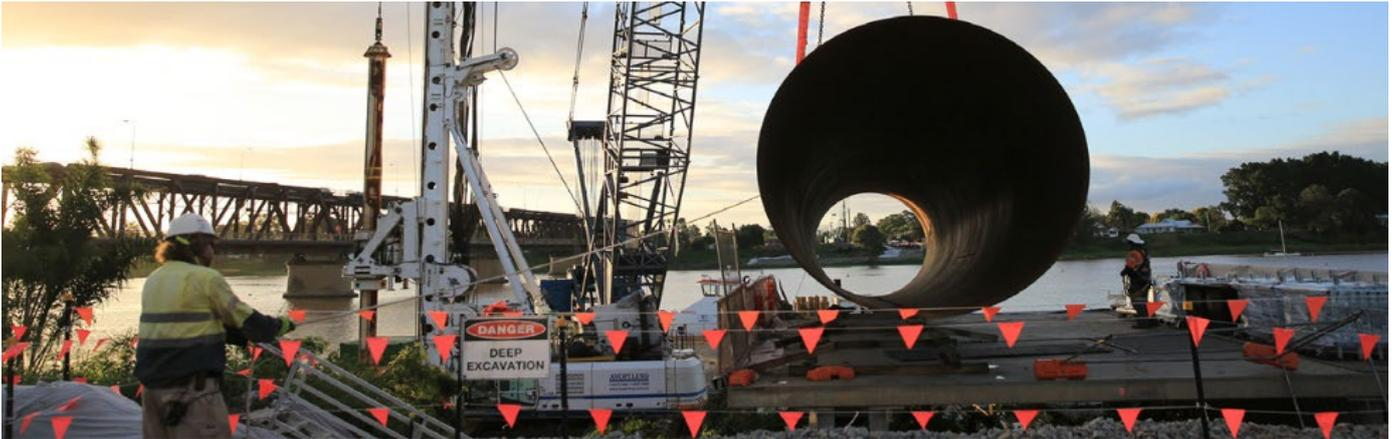
Temporary jetty required for river-based piling work. Grafton Bridge, 2017.
