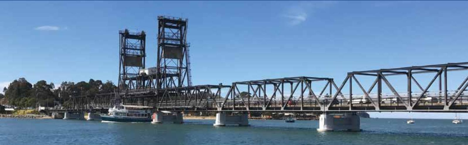
Bridge lift span opening for boat to pass underneath
