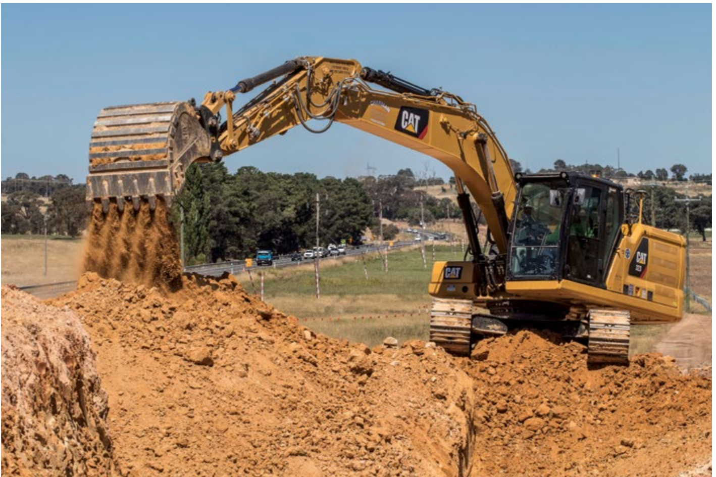
Bulk earthworks under way for the new northbound carriageway
