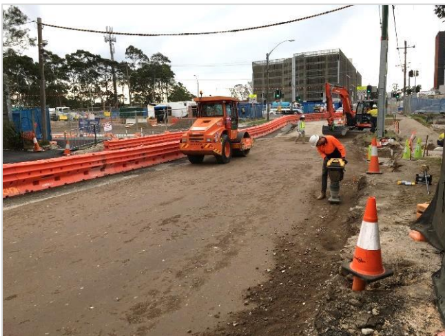
Image: road compaction
