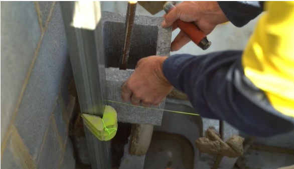
Picture: Installation of the interior block walls
