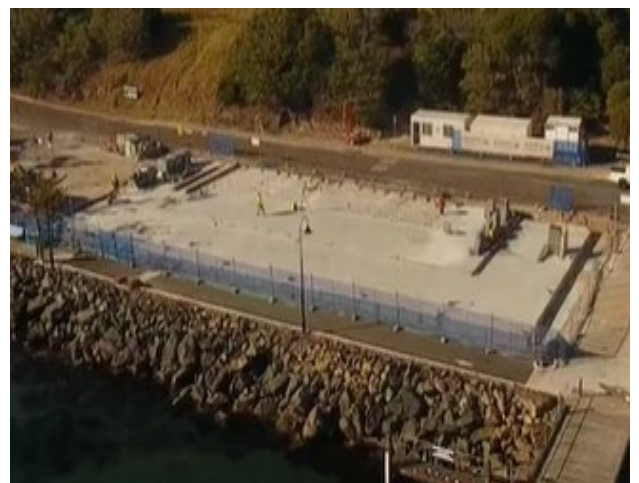
Picture: Aerial view of the Eden Welcome Centre main floor slab
