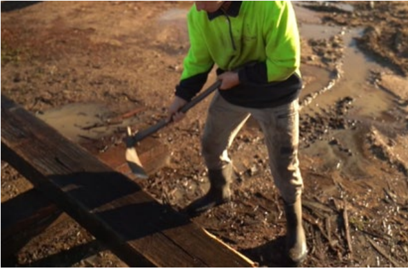
Picture: Preparation of the structural timbers
