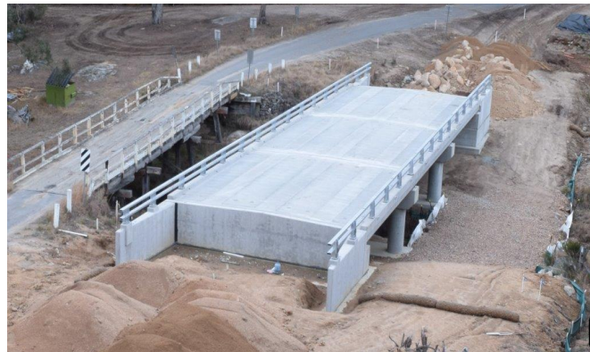
The new Bookookoorara Creek bridge.
