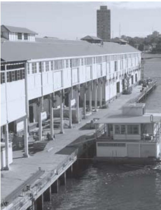
*The refurbishment of Walsh Bay Pier 2/3 continued during the year and comprised replacement of worn piles and substructure as well as the roof and wall cladding*
