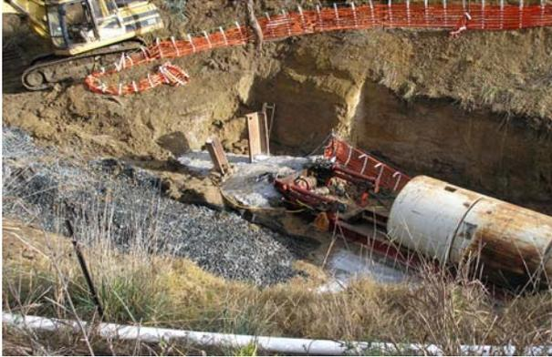
Pipe jacking is a method of installation, which uses jacks to force a specially designed type of precast concrete pipe through the soil. The process may be assisted by removal of material at the leading end via the pipe, using tunnel boring machines, augers or other methods.
