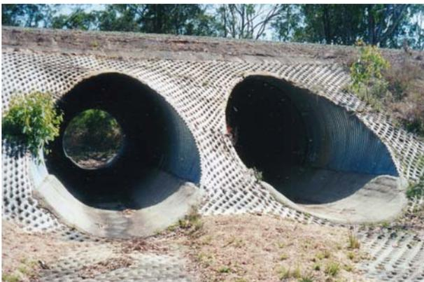
If the corrugated steel culvert is in reasonable condition above the invert area but is eroded in the invert area a new/replacement concrete invert may add several years to the life of the structure. Generic designs have been produced for new or relatively undamaged corrugated steel culverts but site specific designs should be provided where heavy erosion or perforation of the invert has occurred.
