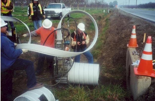
These liners are formed by spirally winding a continuous strip of plastic into the deteriorated corrugated steel culvert and locking or welding the edges of the strip together to form a pipe. Pipes between 150 and 3000 millimetres nominal diameter can be formed in this way.
