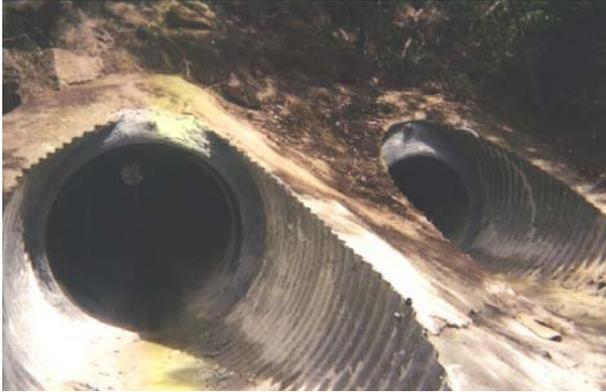
Slip lining involves inserting a high density polyethylene (HDPE) pipe into the steel culvert. Joints are butt welded outside the corrugated steel culvert before being pushed or pulled into place along timber or plastic rails.
