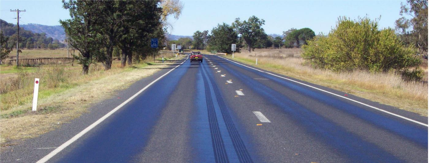
Figure 1: View of a bleeding sprayed seal
