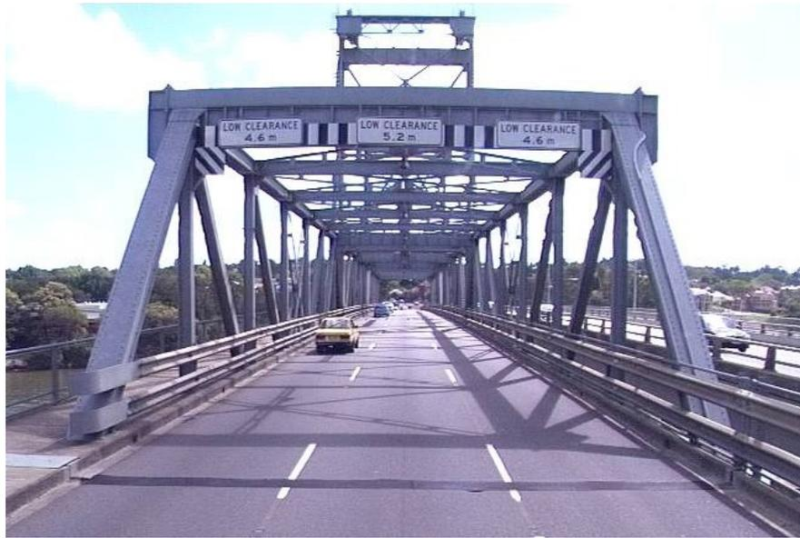
Figure 2007/07 - I - A multi-lane through truss with knee bracings
