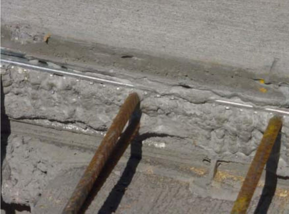
Expanded metal mesh construction joint.
